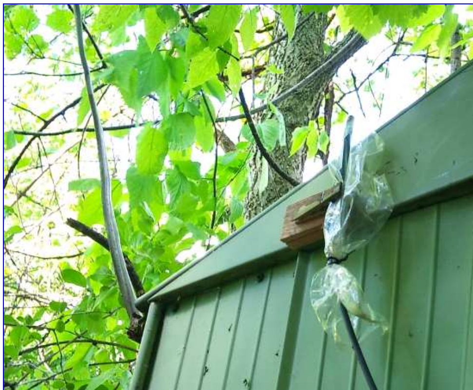
WiFi antenna on the outside of the garden shed for the pool-pump, filter system and the pool timer.
